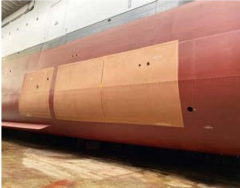
Fig.8: Hull patches coating on Cruise Ship
