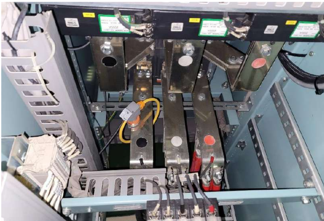
Fig.2: Retrofitted Energy Measurement Device (Rogowski Principle)
