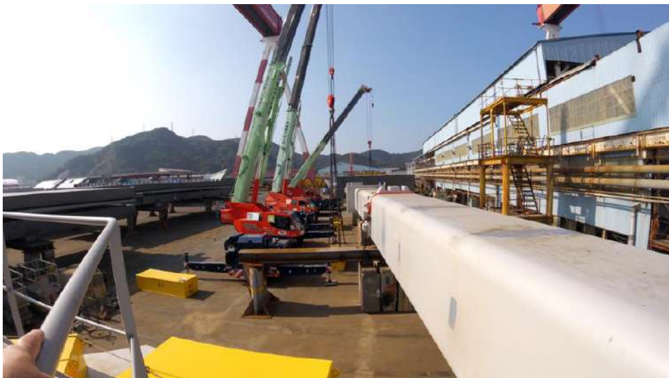
Fig.14: Load test carried out by Class Surveyor for strength verification
