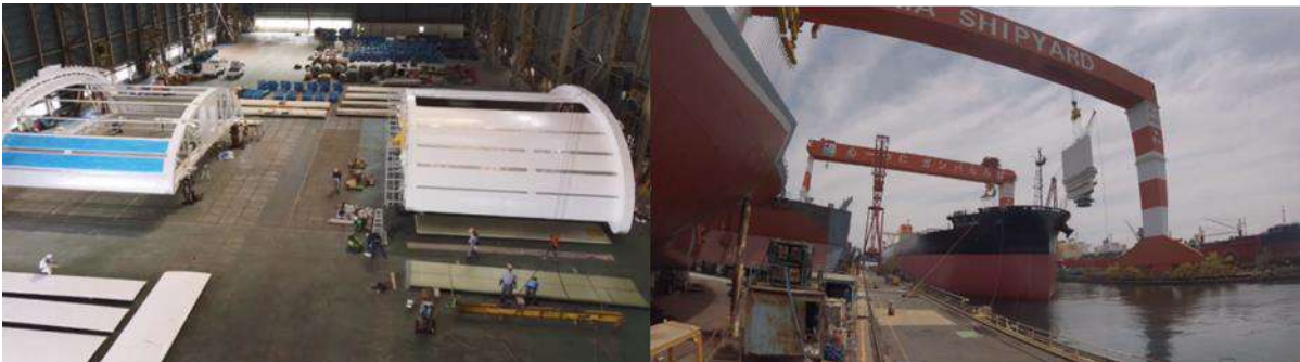
Fig.13: Wind Challenger construction for Shofu-maru
